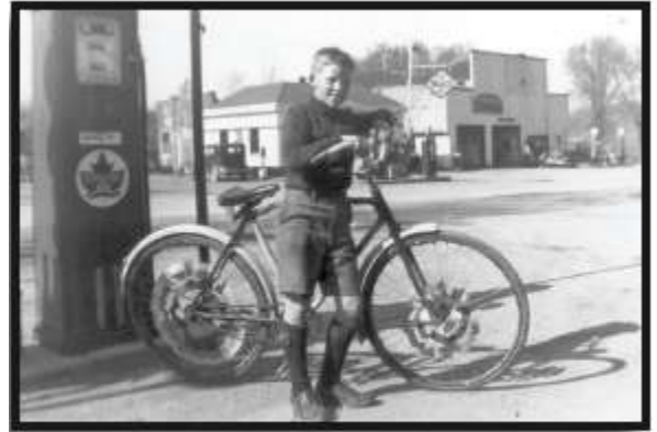
Pump with view of Garage at 12 Elizabeth Street – Doug Pearsall – circa 1940
